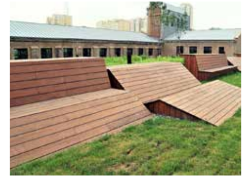
Reconstruction of Jilin Waterworks
